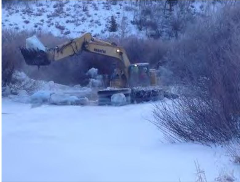
*Figure 13. This photo shows an excavator clearing massive, stratified, apparently dense ice accumulations from Flat Creek. The photo location, date, and photographer are not known.*
